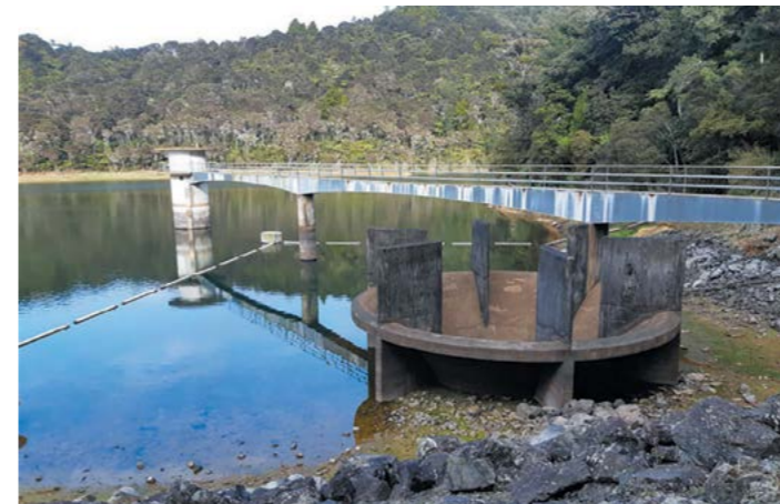
Whau Valley earth dam, Whangārei
